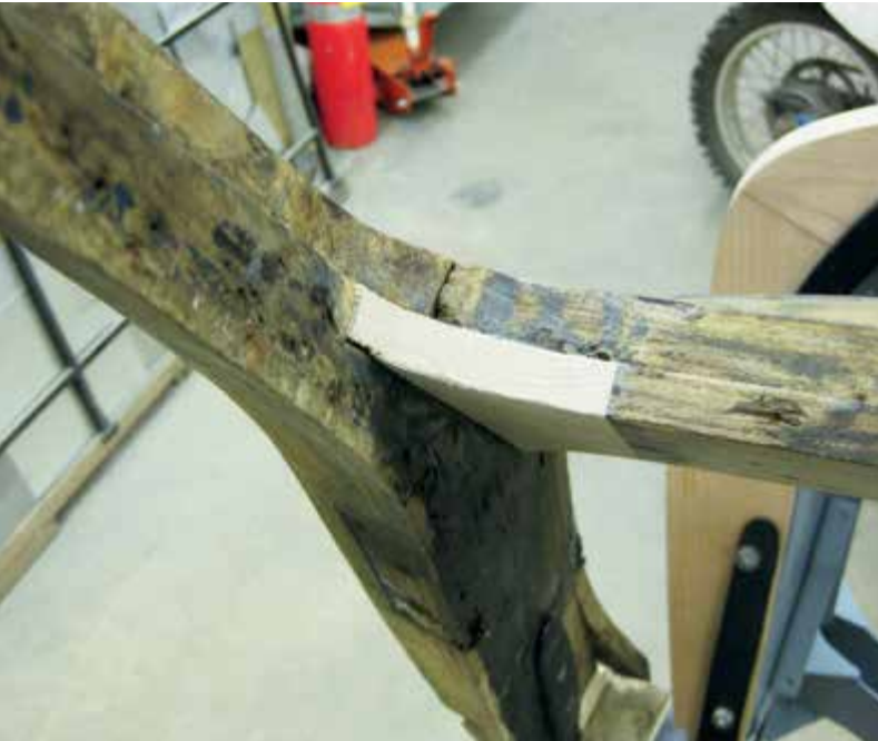
Above: The badly aged wood is replaced while most of the original wooden structure is stabilized and saved.
